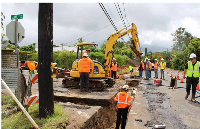
Hanalei Waterline project construction
