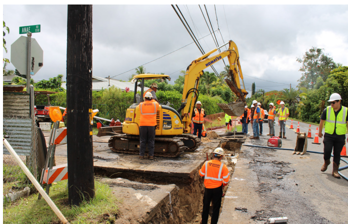
Hanalei Waterline project construction
