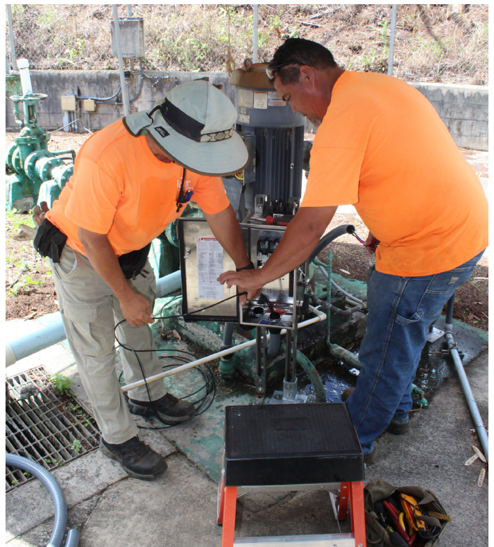
KDOW electrical plant staff work on improvements to a pump station
