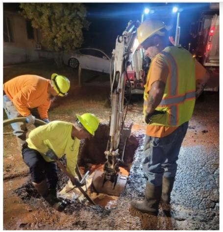
Water Department workers inspect and repair a damaged pipe that provides water to homes and businesses from the water main. (Courtesy: Kauai Department of Water/2023)
